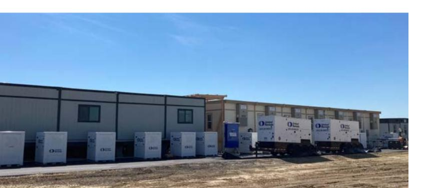
In many cases, a BESS is a standalone unit that can connect with a generator or provide power on its own. The POWRBANK is one example. The model offered by United Rentals is rated for 40kW to 60kW of power output—enough to power a guard shack overnight—and provides between 60kW and 120kW hours of storage. Other products, such as the ANA Energy Boss, provide all-in-one continuous power, with the BESS, generator and control systems housed in one unit.
