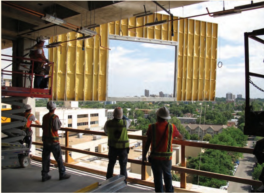
Installation of a prefabricated exterior wall panel.
