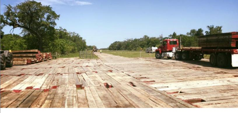
For long projects, temporary gravel engineered roads may be an option for vehicle traffic, but they are expensive and time-consuming to build and remove. Construction access mats can save time and money in comparison.
